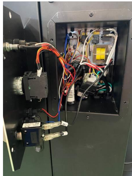
Figure 8: Control Panel/Box Wiring
